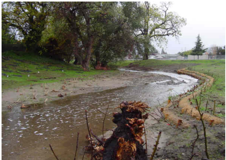
Mission Creek with coir logs to the right to protect erosion of the bank.
