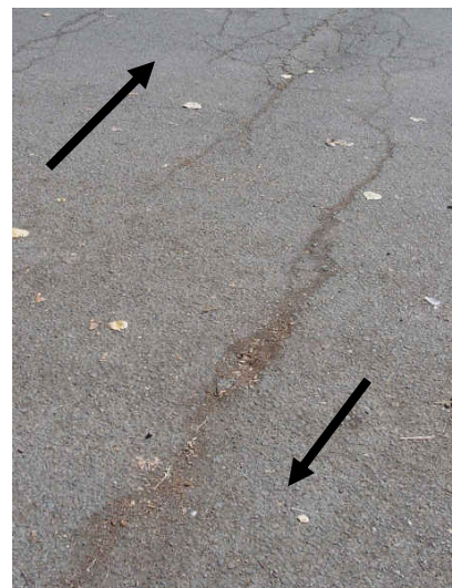
En echelon fault pattern seen in the asphalt
