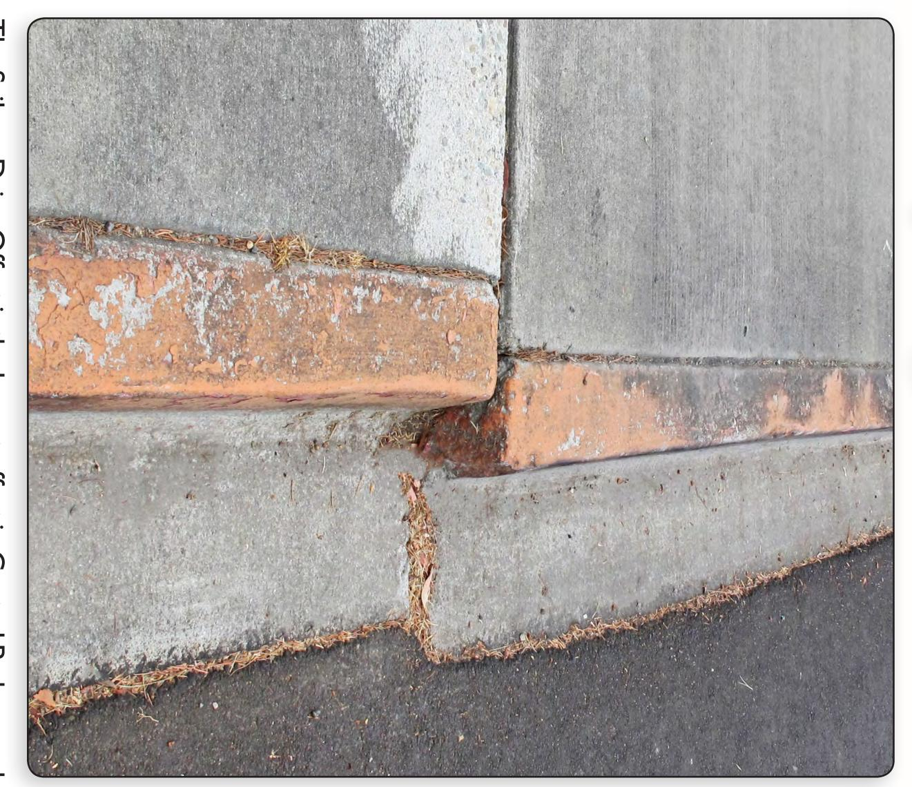
The Sailway Drive Offset is the largest offset in Central Park caused by tectonic plate movement along the Hayward Fault. The curb has a dramatic shift of greater than 3 inches caused by a strike-slip fault movement.
