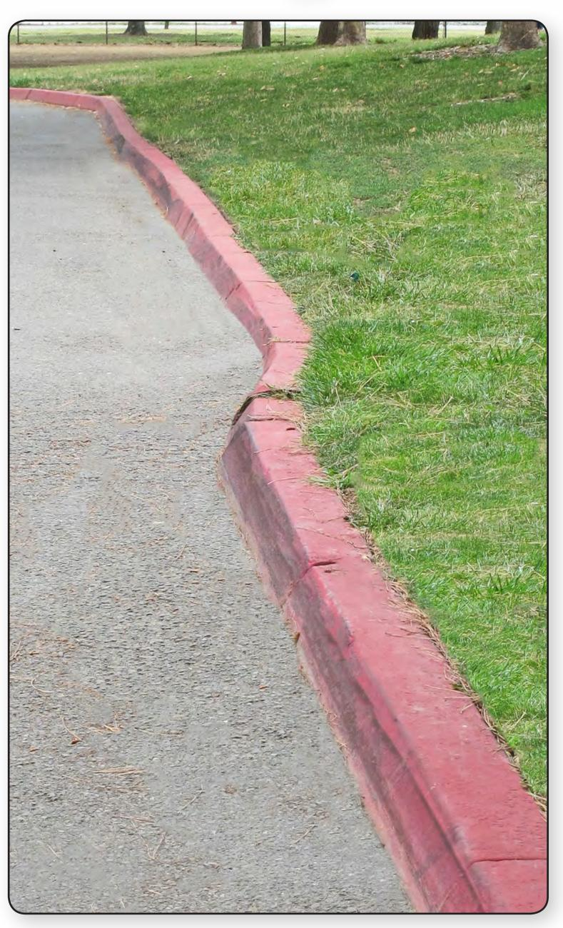
While at Central Park keep an eye out for evidence of fault movement. In this parking lot, the Hayward Fault is causing linear breaks in the asphalt and concrete curbs. The rate of movement, around 5 millimeters per year in the Fremont area, is enough to visibly move structures within a few years.
