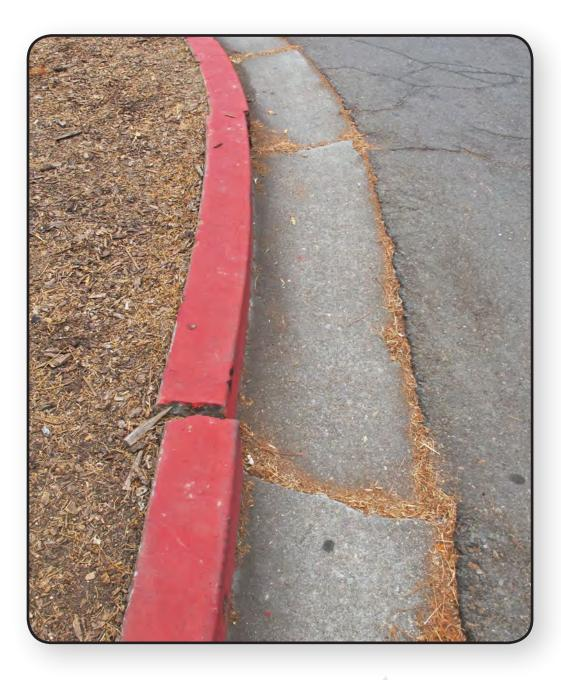
The offset of the curb is dramatic, showing a shift of an entire area. This is one of the most impressive of the offsets because it visually shows evidence of movement.
