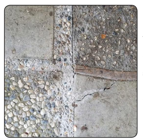
Wood and concrete react differently to constant fault creep. Look at the wood strips between the concrete and notice the wood is bending. As the wood bends, the concrete will crack.
