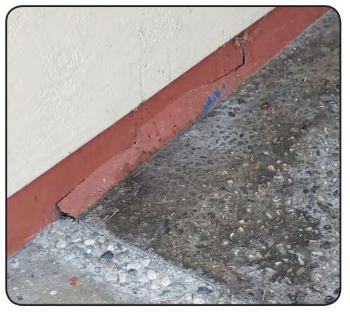
The inside of the building shows evidence of accumulated movement since the building was constructed in 1962. Outside, the patio has also slowly shifted as seen in the concrete.
