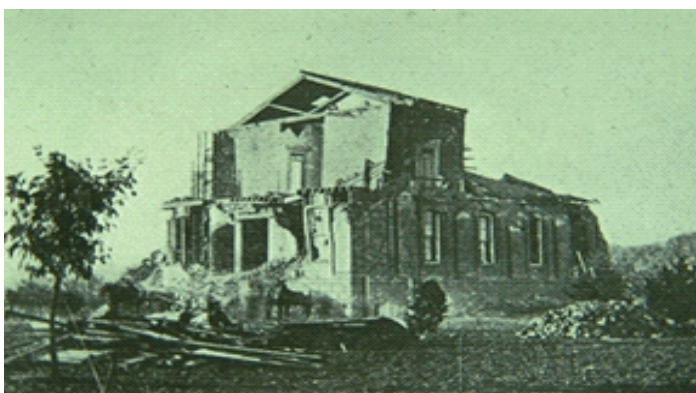
Court house in San Leandro collapses after 1868 earthquake
