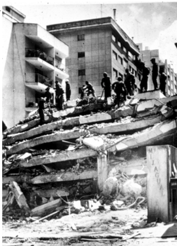
Building collapse caused by earthquake shaking, Caracas, Venezuela
