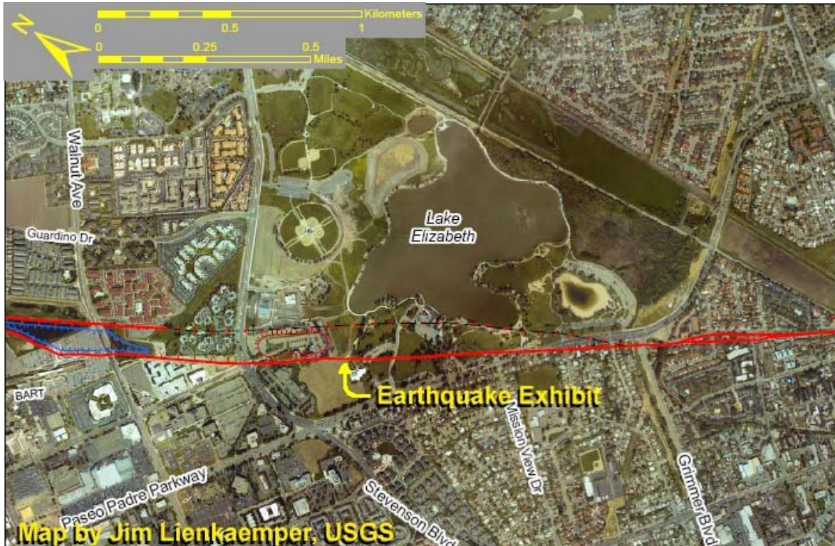
Area of walking Tour including Tyson Lagoon on the left, present site of Earthquake Exhibit and Stivers Lagoon on the right.
